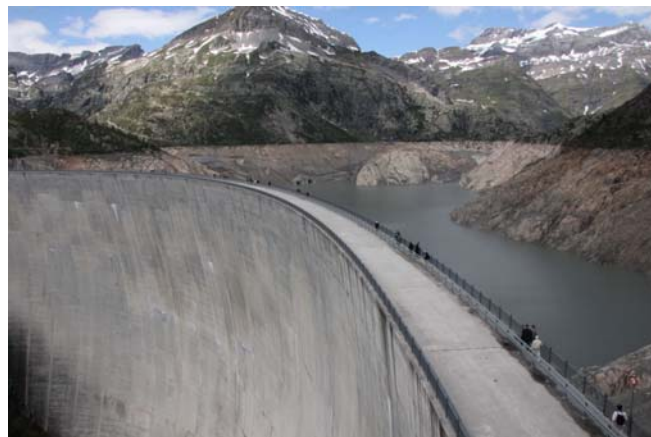
The Nand-de-Drance (Switzerland) pumping-storage scheme is using the Emosson dam as lower reservoir.
