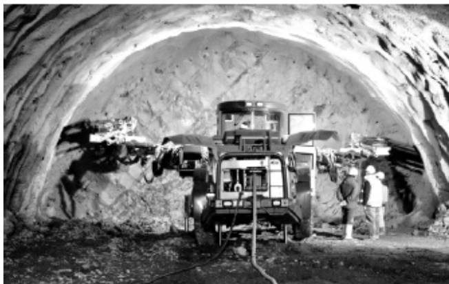
Figure 9: Sandstone and siltstone molasse exposed in the face of a 12 m span tunnel top heading in Greece.
