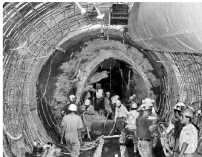
Figure 16: Failure of a tunnel section due to very severe squeezing (background) and re-mined and re-supported tunnel (foreground).
