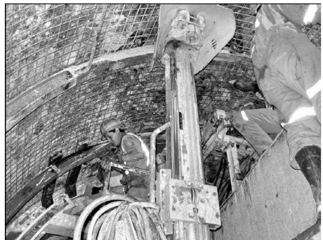
Figure 8. Installation of steel sets immediately behind a TBM shield in the Olmos tunnel in Peru. Photograph provided by R. Guevara (2008).
