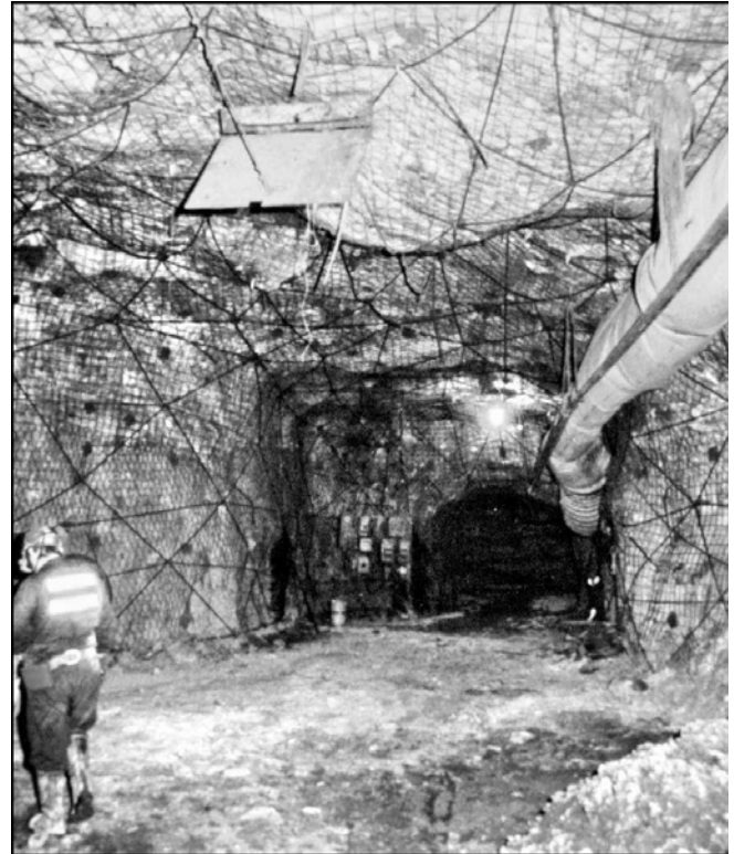
Figure 7. Cable lacing in a deep level hard rock mine to control damage from brittle failure. Tensioned cables are attached to grouted anchors installed on a regular pattern.
