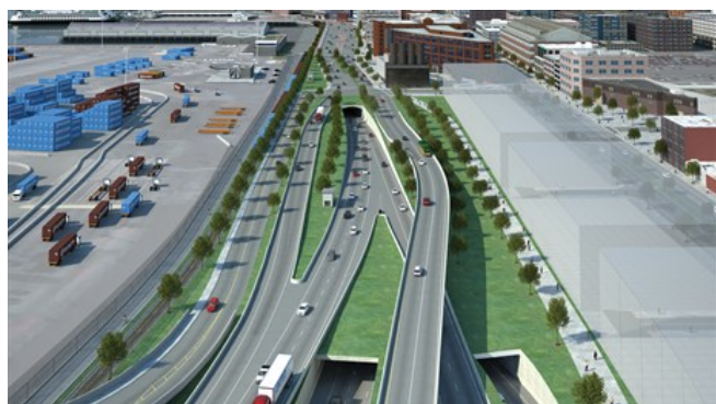
Ramps and cut and cover tunnels at the tunnel approaches will feed traffic into double deck formation
