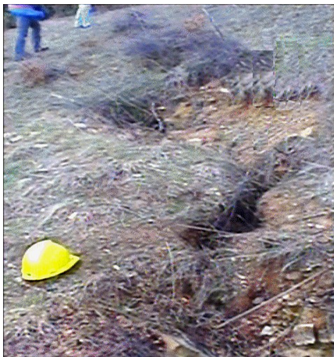
Figure 21. Extended tensional cracking of the ground surface upstream on the hill.
