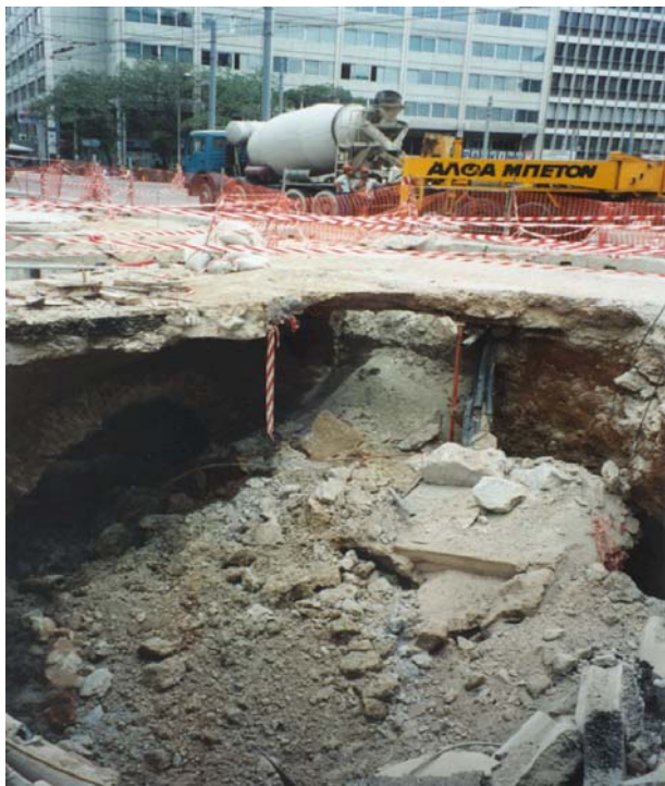
Figure 11. Significant over-break failure at Aghiou Konstantinou street. Athens Metro project.
