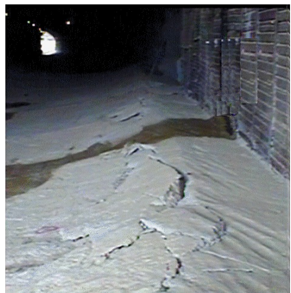
Figure 20. Significant cracking of temporary invert.
