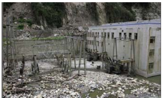
Figure 6. Damage of Shapai powerhouse due to rockfalls and flooding (up) and sediments from flooding due to penstock failure inundating the powerhouse and switchyard (down) (Wenchuan earthquake, China).
