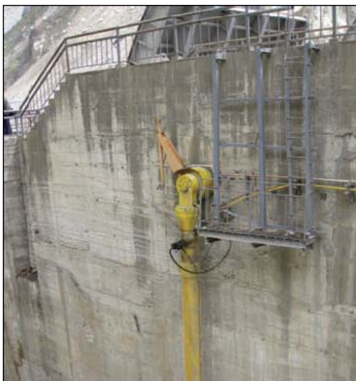
Figure 4. Failure of radial gate of Taipingyi weir due to rock-fall (Wenchuan earthquake, China): Intact radial gate (up), and hydraulic piston of failed gate (down).
