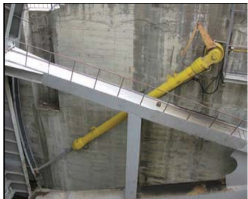
Figure 3. Damage of gate of power intake due to rockfall (Wenchuan earthquake, China).
