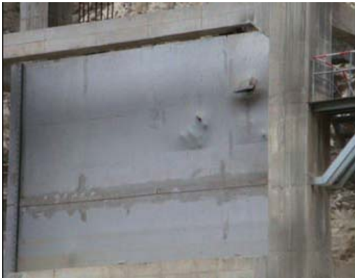
Figure 3. Damage of gate of power intake due to rockfall (Wenchuan earthquake, China).
