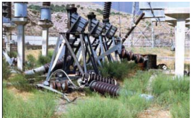
Figure 5. Failure of transmission tower caused by rockfall (up) and failure of switchyard components caused by ground shaking and settlement of fill material (down) (Sefid Rud dam; 1990 Manjil earthquake, Iran).
