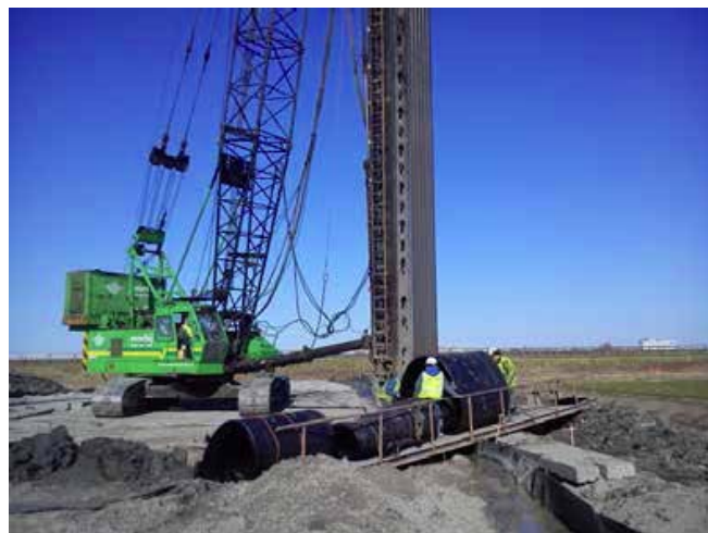
Photo 2 Installation of a membrane wall in Leeuwarden, Netherlands - Source: Combination Grutte Fier (Mobilis, De Vries, Van Gelder and Oosterhof Holman).
