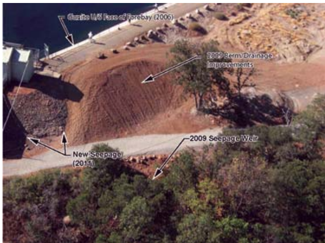
This photo shows the location of the seepage at the Hat Creek No. 1 forebay embankment, as well as where the new berm was built to prevent seepage.
