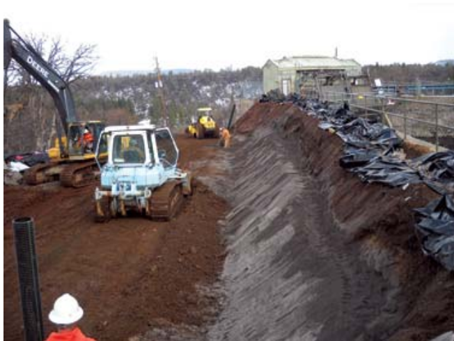
A new, wider, and more stable embankment was constructed at the Hat Creek No. 1 facility once the sub-drainage system was installed.
