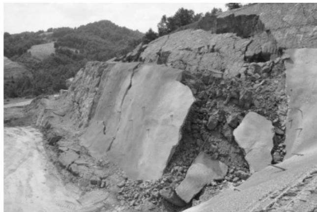
Figure 3. Landslide in molassic formation at the entrance portal of the Karatzas tunnel in Egnatia Odos.
