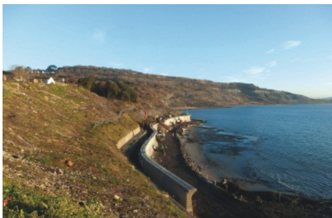
Coastal protection: The haul road provided access and protected the World Heritage rock ledges
