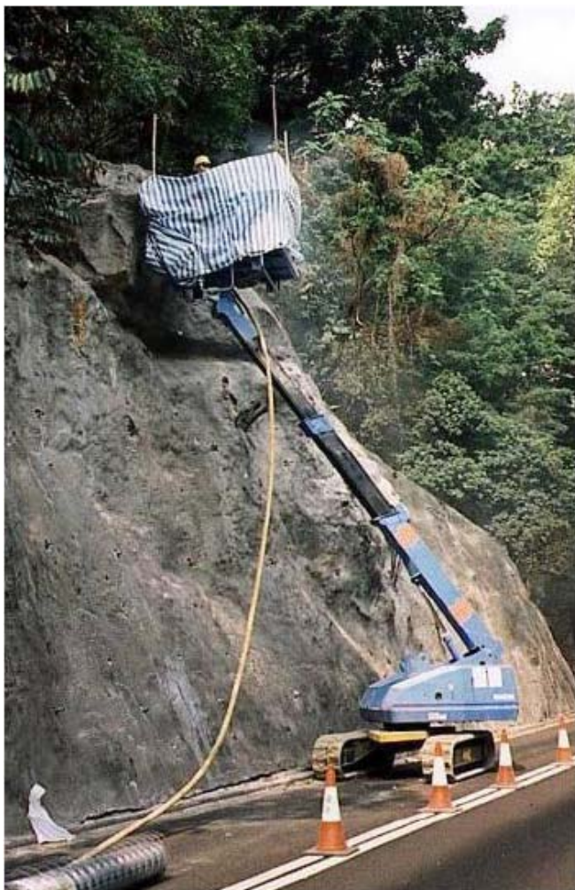
Figure 7. Mobile Platform for Soil Nailing Works
