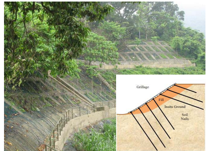
Figure 5. Use of Soil Nails to Stabilize Fill Slopes
