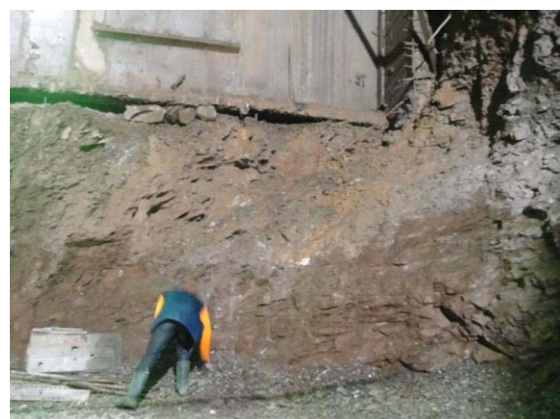
Distressing of the siltstones after excavation, under the concrete struts
