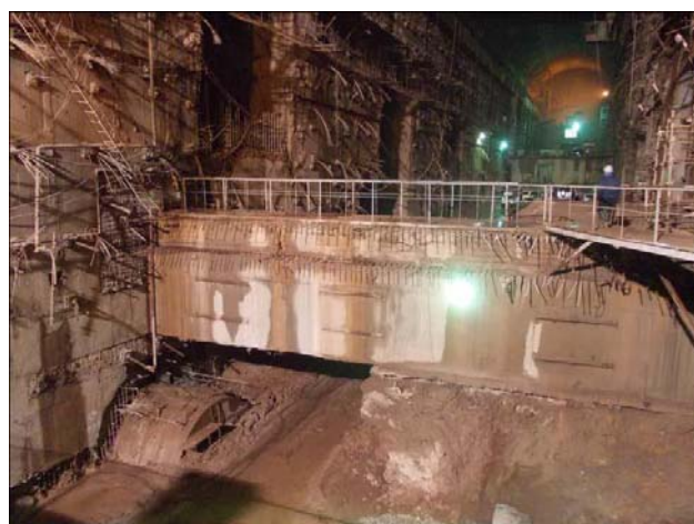
Placement of struts to face deformations
