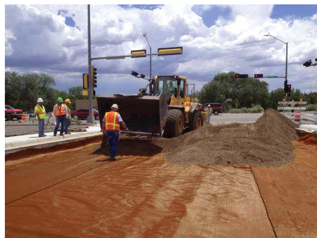
A new wave of geotextiles, such as TenCate's Mirafi® RSi series, are characterized by exceptional strength and reinforcement performance. Photo by TenCate Geosynthetics Americas.
