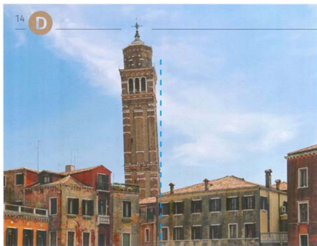
Land subsidence in areas with soft soil, like those in and around Venice, can, in combination with poor foundations, result in the subsidence of historic buildings, as here in the case of the Santa Maria Gloriosa del Frari.
