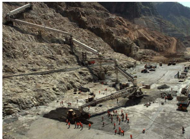
First RCC placed at Gibe III on 18 December, 2011
