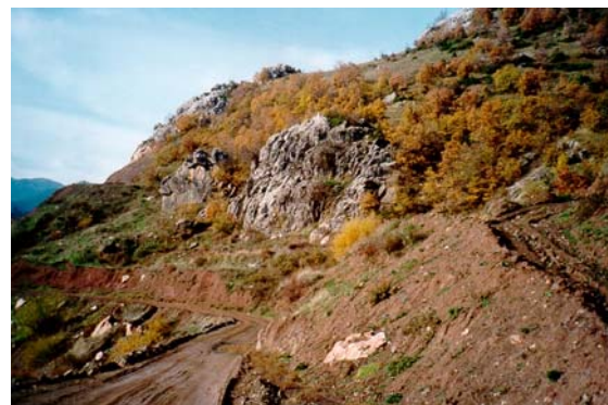
Figure 4: Blocks in melange protrude from hillside along proposed right-of-way, Egnatia Highway, Greece. (Photo: late Professor Gunter Riedmueller/GGG, Austria)
