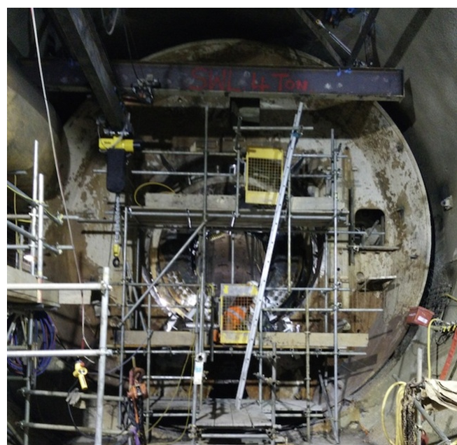
The cutter head of TBM Elizabeth, which is slowly being broken apart and removed from the tunnel.
