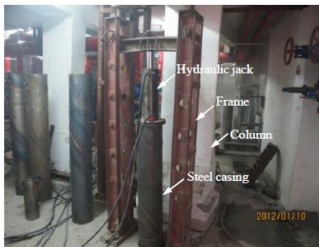
Figure 11. Underpinning column foundation with jack-down piles
