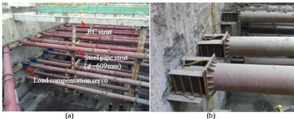
Figure 10. (a) Load compensation servo for steel struts; (b) close-up of the connection between retaining wall and the servo
