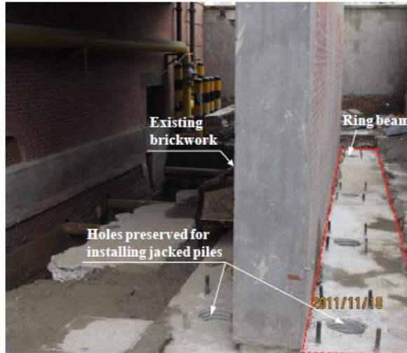
Figure 12. Underpinning brick wall foundation with pile and beam
