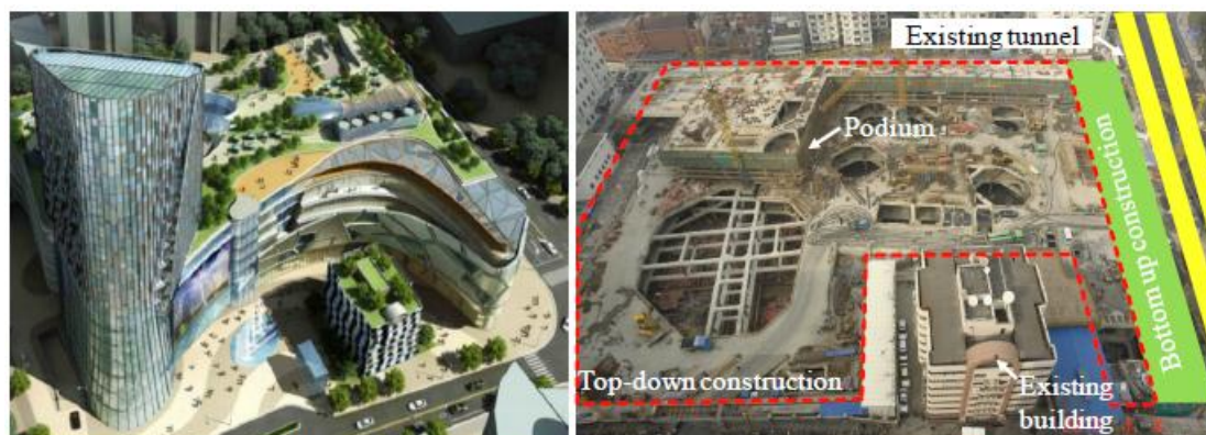
Figure 7. Excavation of Jing'an transportation hub constructed using concurrent upward and downward method (excavation area=16000 m 2 , excavation depth=17.2 m)
