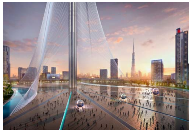
Structural core and tension cables disguised as delicate ribbing of lily leaves anchor the building to the ground.
