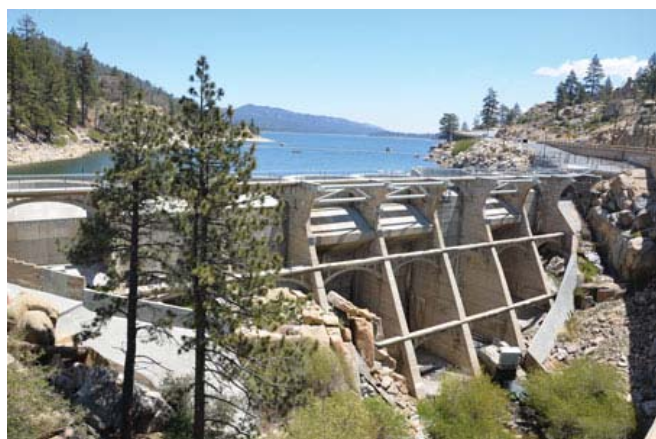
Bear Valley Dam is a 92-foot-high multiple barrel arch dam in southern California. Work to ensure the spillway gates were ready to operate was required in the event of a large rainfall event from El Nino.
