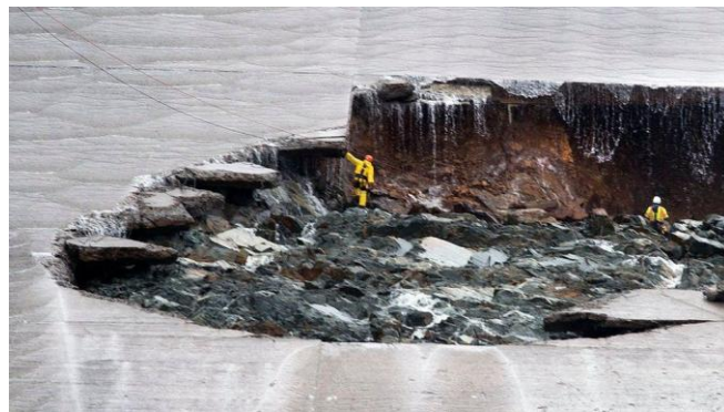
Workers inspecting a damaged part of the Lake Oroville spillway earlier in the week
