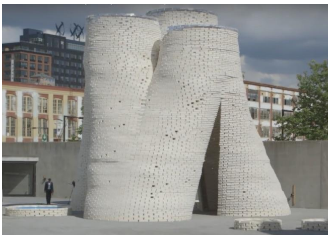
Building a 40-Foot tower made of living mushroom bricks
